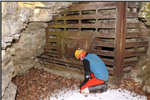
*Installed in 1986, the former gate at Horseshoe bay cave restricted air flow and was not compatible with current bat-friendly gate standards.*
